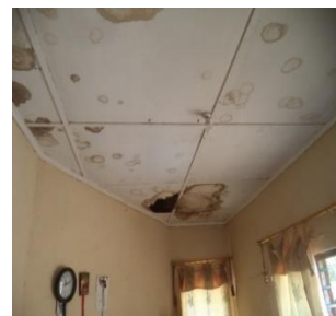
Dilapidated ceiling board at the Visitor Information Centre at Chishimba Falls
