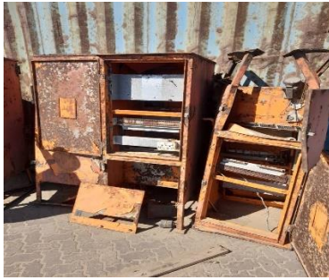
Part of the Stripped non-functioning plug point That used to connect 96 refrigerated Containers
