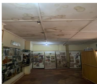
Dilapidated ceiling board at the Visitor Information Centre at Chishimba Falls
