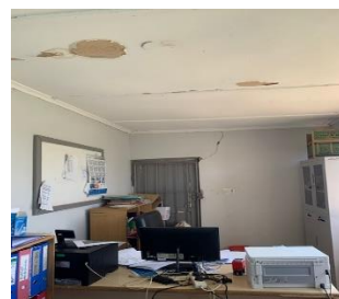
Dilapidated ceiling board and cracked wall plate at the Kasama Regional Office
