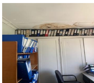
Dilapidated ceiling board and cracked wall plate at the Kasama Regional Office
