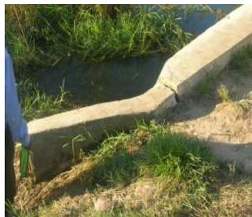
*A crack on the culvert head*
