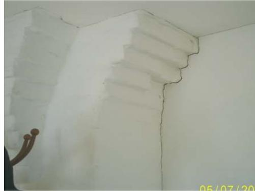
*Peeling paint on the wooden walls and cracks between wooden walls and pillars*
