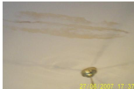
*Peeling paint due to leaking roof*
