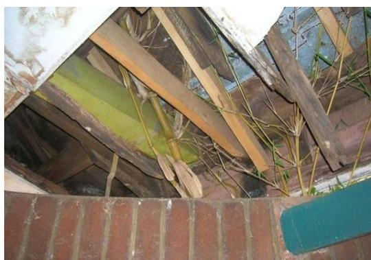
*A roof at the servants quarters damaged by a bamboo Plant.*
