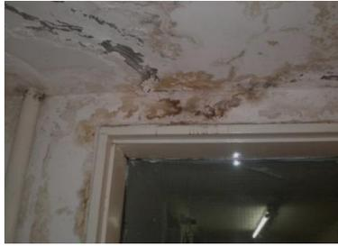
*Part of concrete ceiling showing leakages*
