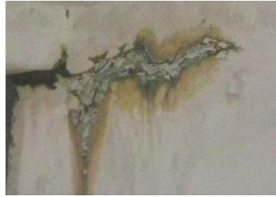
*Cracks on the wall showing leakages*
