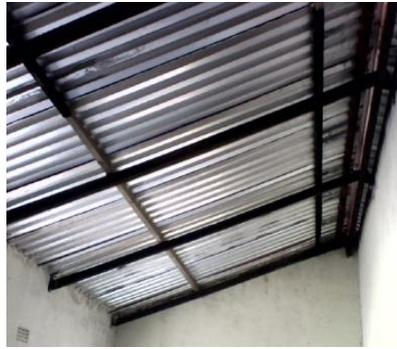
*No trusses in the roofing.*
