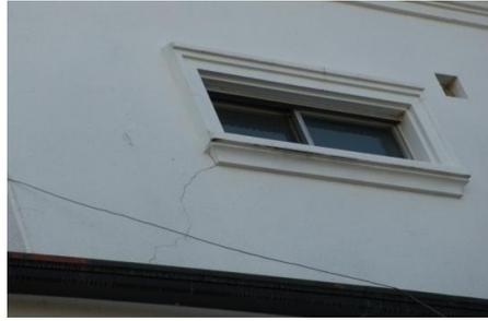
*Cracks in the wall inside and outside the house*
