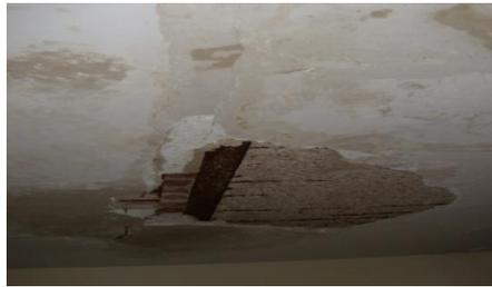
*Cracked and falling concrete roof*
