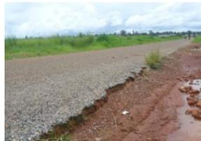
*Road surface dressing being eroded from the Solwezi College Road due to lack of a drainage system*
