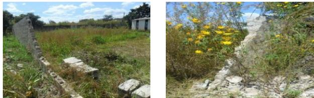
*A collapsed section of the rehabilitated wall fence at the Solwezi Stadium Complex*
