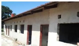
*Window frames, doors, air vents and window panes not fitted*
