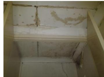
*Damaged ceiling due to leakages*
