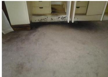
*Damaged floor due to leakages*
