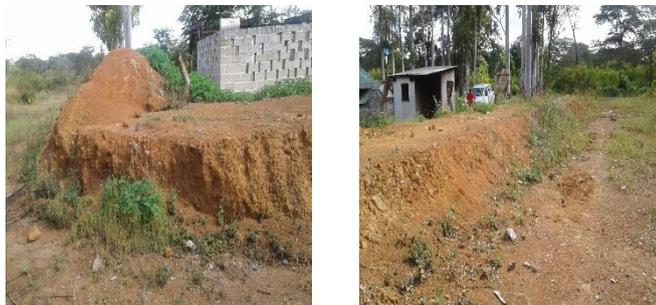
*Unrepaired Collapsed Embankment at River Water Pump Station in Mufulira*
