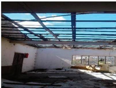
*Part of Building with Blown off Roof.*
