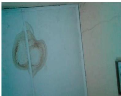
*Warehouse with damaged ceiling board due to leakages*
