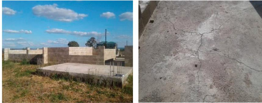
*Incomplete Provincial Local Court Office Block with Cracks on the Slab*
