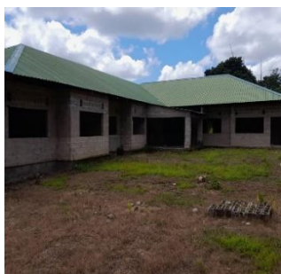
Stalled works - front view
