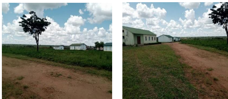
Section of eight (8) prison cells not Operationalized
