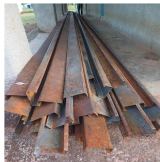
Unutilized roofing materials
