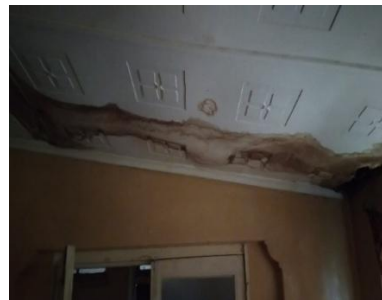
Damaged roofing and ceiling board
