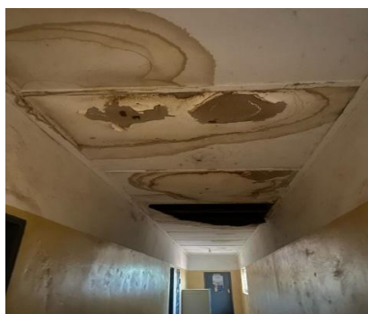
Stained Ceiling due to Leaking Roof
