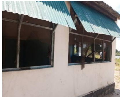
Damaged ceiling board, broken windowpanes and cracked wall
