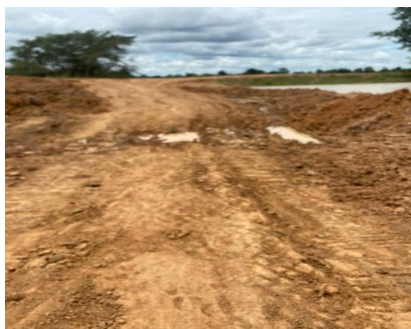
Mauka dam Maintenance
