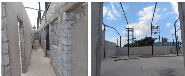
Construction of the Warehouse at Roof Level
