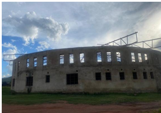
Incomplete Roofing on Theatre Hall
