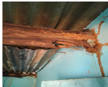
Broken trusses
