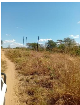
Poles without cables
