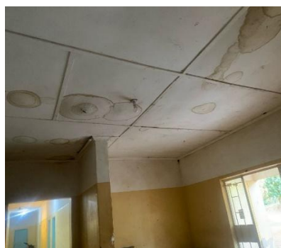
Stained Ceiling due to Leaking Roof
