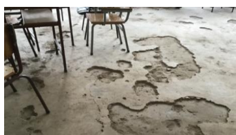
Disintegrated floor
