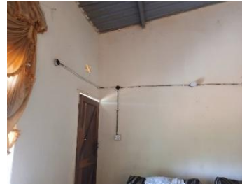
Door not fitted at Chiendeyende Improvised electrical fitting at Mphuka
