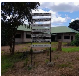
Stalled works - front view
