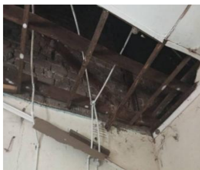
Damaged ceiling board, broken windowpanes and cracked wall
