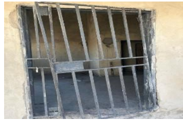
Poorly fitted grill door
