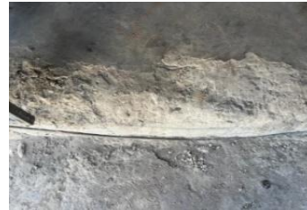
Eroded floor
