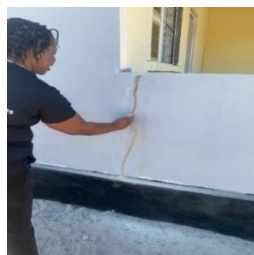
Cracked walls
