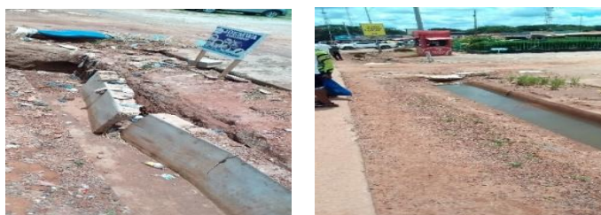
Collapsed pavement and culvert walls
