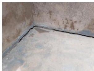
Crack between the floor and the wall Incomplete 1x3 classroom block
