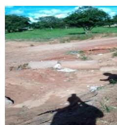
Road eroded and had developed potholes
