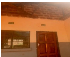
Ceiling board and electricals not installed
