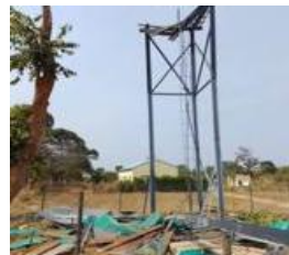
Broken water tank and damaged solar panels Collapsed water reticulation system
