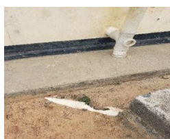
Worn out paints Broken sewer pipe Missing inspection cap
