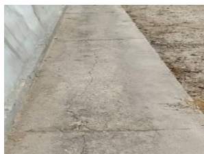
Cracks on the apron
