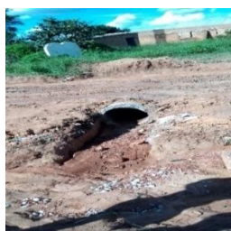
Road eroded and had developed potholes
