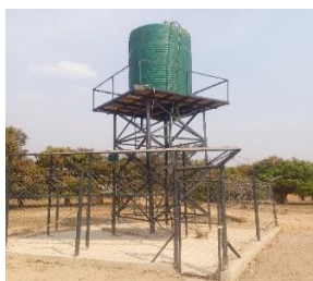
10,000 litres tank installed instead of 20,000 litres tank
