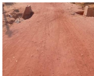
Inlet and outlet head had been eroded.
