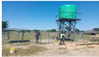
Incomplete solar powered borehole
