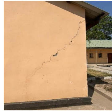
Crack - Exterior Wall of the Council Chamber
