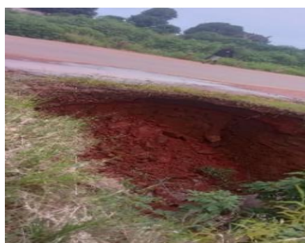
Eroded side drain
