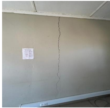
Crack - Old Engineering Office
