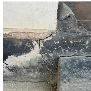
Cracks - Foundation of Building
