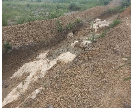
Section of the drainage with Unblasted Rocks
