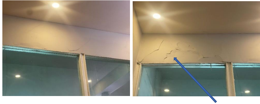
Cracked Boards in the Foyer
