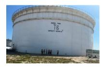
Rehabilitated Tank 6 without Concrete Works on Bund Surface Area
