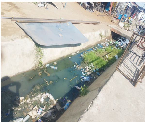
Figure 6.6: Clogged, Uncleaned Drainage with Grown Grass in Chawama and along Mumbwa road in Lusaka.
