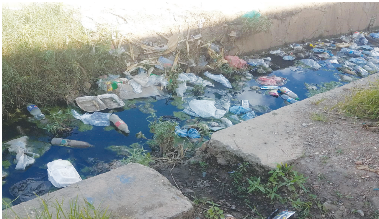
Figure 6.13: Drainage filled with Solid Waste in Chawama.
