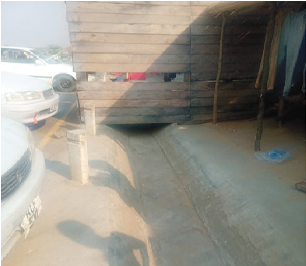
Figure 6.10 Makeshift Shops Constructed on the drainage line in Sioma.
