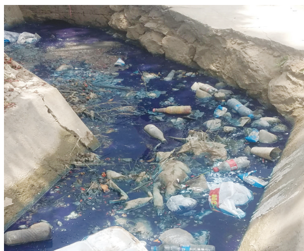
Figure 6.6: Clogged, Uncleaned Drainage with Grown Grass in Chawama and along Mumbwa road in Lusaka.
