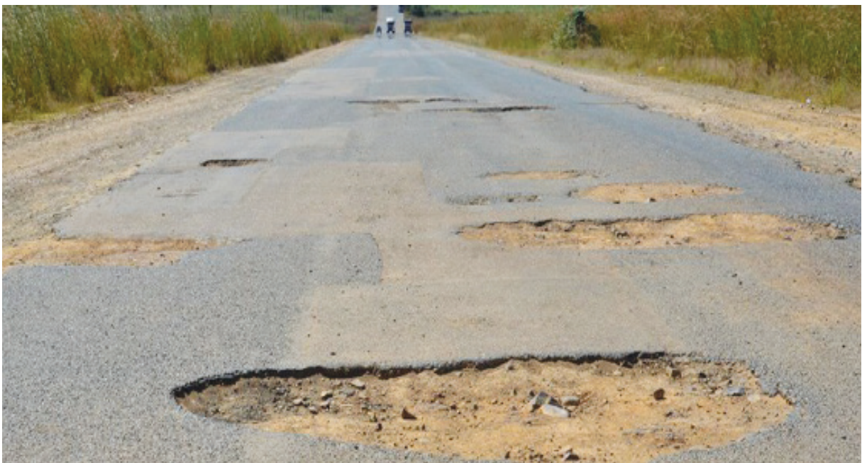
Figure 6.14: Lusaka-Ndola Road riddled with potholes.
