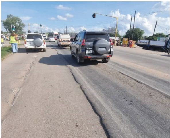
Figure 6.21: Longitudinal cracks and alligator cracks on Luangwa-Nyimba Road
