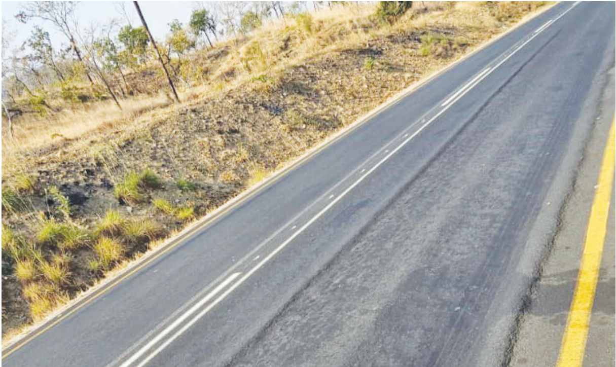
Figure 6.13: Road rutting between Nyimba and Luangwa bridge
