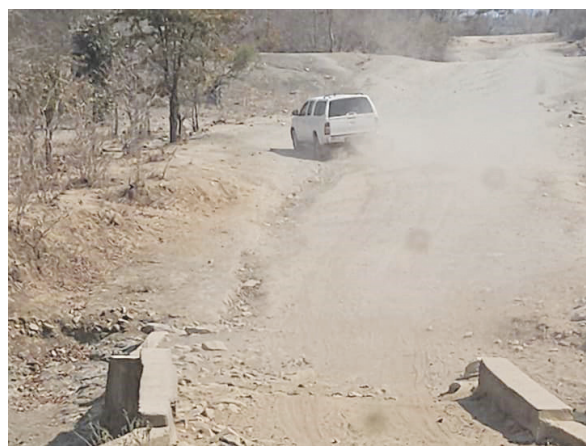
Figure 6.27: Gwembe to Bottom road with corrugations and in general poor condition.
