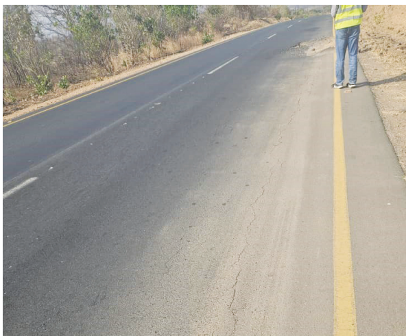
Figure 6.21: Longitudinal cracks and alligator cracks on Luangwa-Nyimba Road
