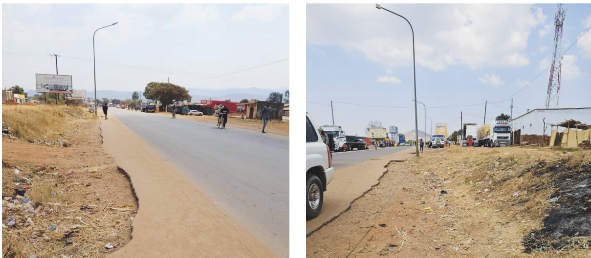
Figure 6:28: Eroded road shoulder due to HGVs - Mchinji Border Station in Chipata
