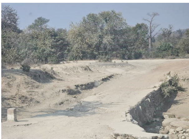
Figure 6.27: Gwembe to Bottom road with corrugations and in general poor condition.
