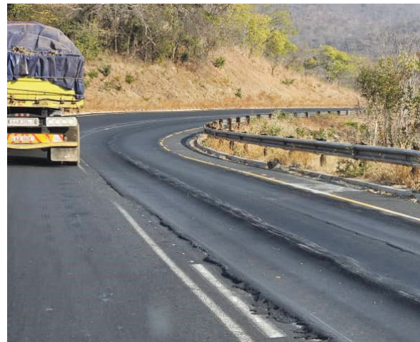
Figure 6.21: Longitudinal cracks and alligator cracks on Luangwa-Nyimba Road
