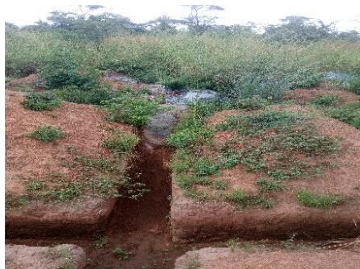
Mpongwe - Foundation for one of 10 medium cost houses
