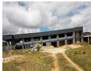
Incomplete Administration Block
