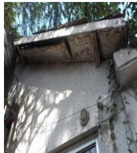
Ceiling board at the Chancery flat Warping ceiling board on the 3 rd floor
