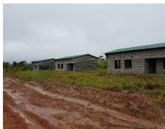
Incomplete low cost staff houses
