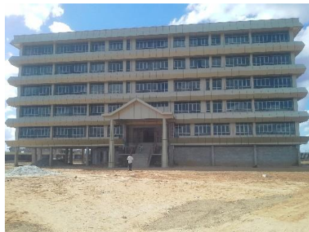
The Exterior Office Block
