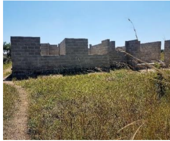
Medium Cost House at ring beam level
