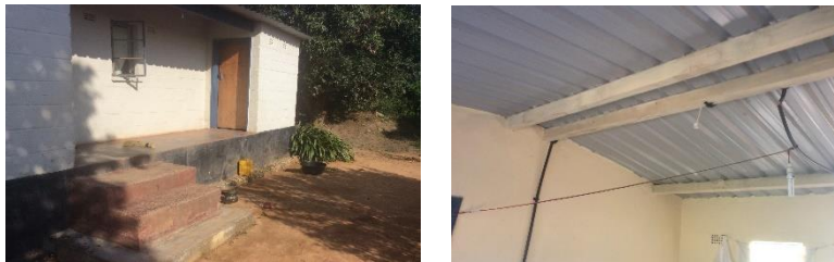
Camp house veranda and internal roofing
