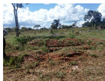
Mpongwe - Part of the foundation for the Post Office
