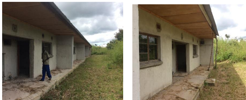
Incomplete Dormitory structure
