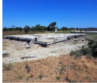
Medium Cost Houses at slab level
