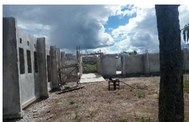
Police post under construction in Mpongwe
