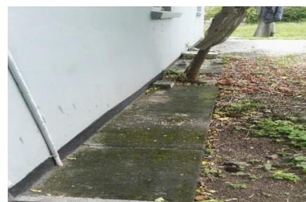
Part of the apron done for House No.1
