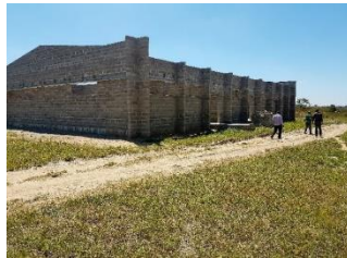
Maternity wing at ring beam level
