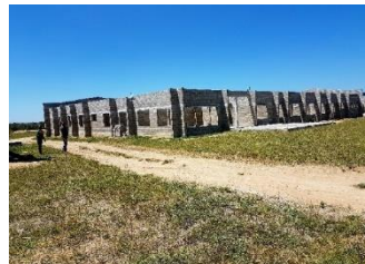
Theatre Block at wall plate level
