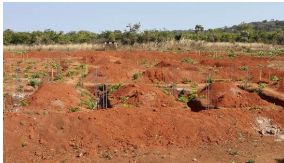
Chinsali Lodge Construction Site
