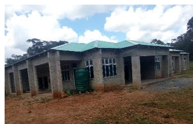
Post office Block under construction in Lufwanyama
