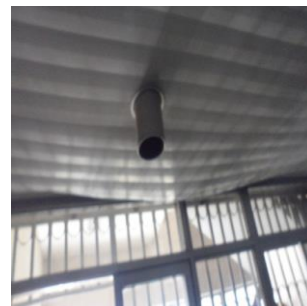
Ceiling board at the Chancery flat Warping ceiling board on the 3 rd floor
