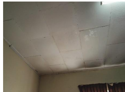
Warping ceiling board
