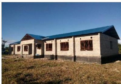
Incomplete Office Block at Fiyongoli Aquaculture Research Station
