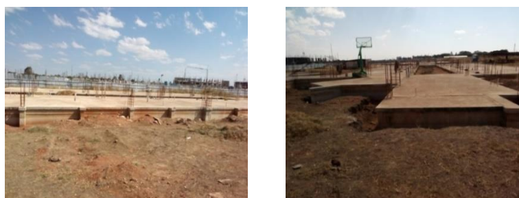
All the Hostel blocks at Slab level
