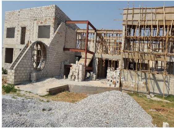
Administration block under construction at National Science Centre
