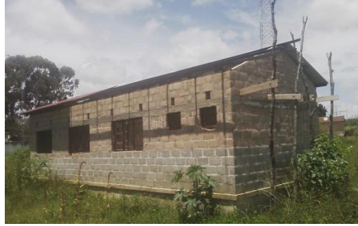
Incomplete Office Block
