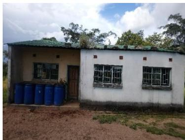
Staff House with broken windows and damaged roof
