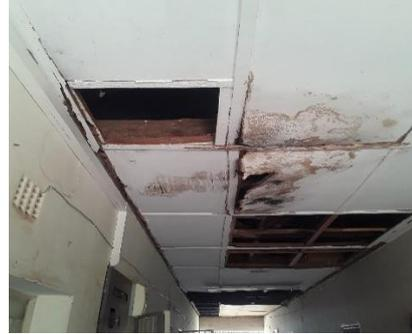
Traces and Ceiling Boards Damaged by Termites
