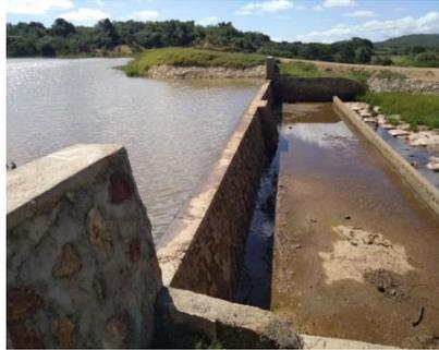
Spillway and embankment requiring raising
