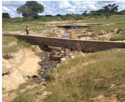
The eroded spillway requiring repairs
