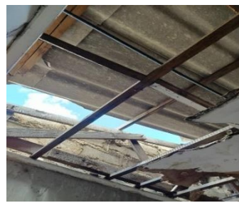
Blown off Roof and Worn out Ceiling
