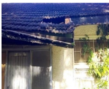
Worn out roof tiles
