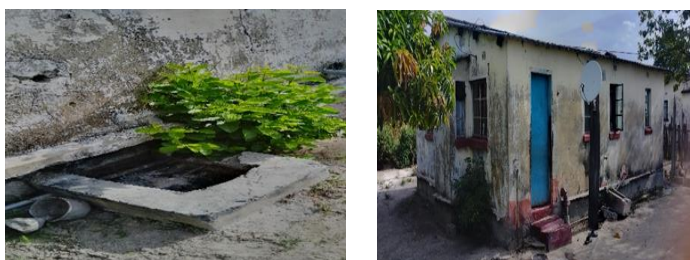
One of dilapidated Staff House and Sewer leakage at Namwala Correctional Facility
