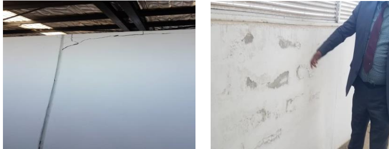
Cracks on the newly constructed walls and paint peeling off on just painted
