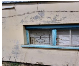
Visible cracks and broken window panes DC's Residence
