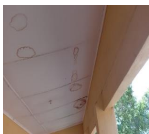
Leaking roof of the administration block
