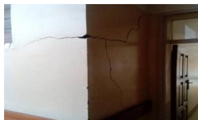
Cracks on the wall of Administration Block
