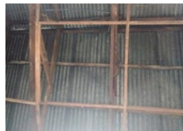
Cell Ceiling without wire mesh
