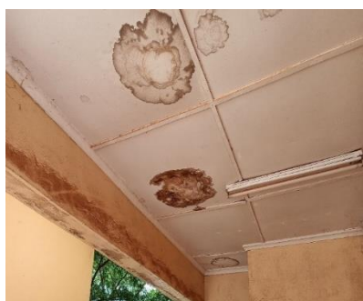
Leaking roof
