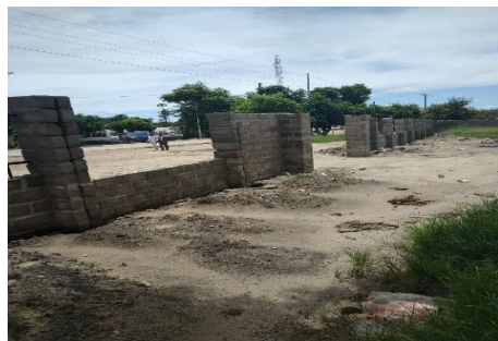
Incomplete wall fence, unplastered and unaligned block works (February and May 2023)
