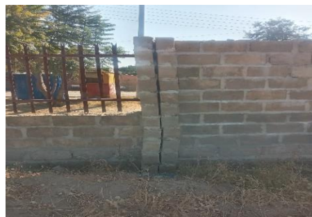
Incomplete wall fence, unplastered and unaligned block works (February and May 2023)
