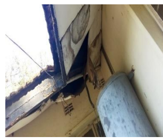
Rotten Ceiling Board
