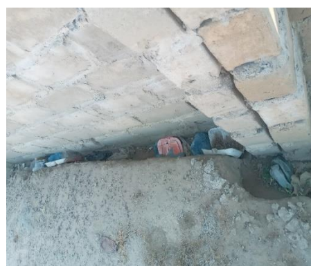
Foundation excavation not fully backfilled
