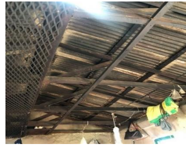
Partial wire gauze and worn-out wire fence
