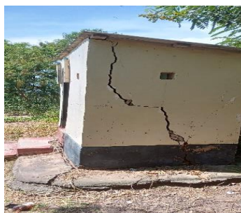
Crack on the VIP Latrine
