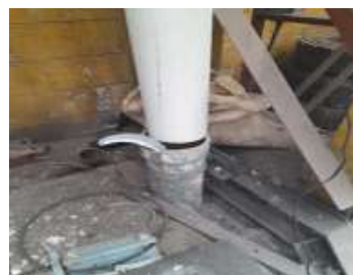
Incomplete Drain pipes
