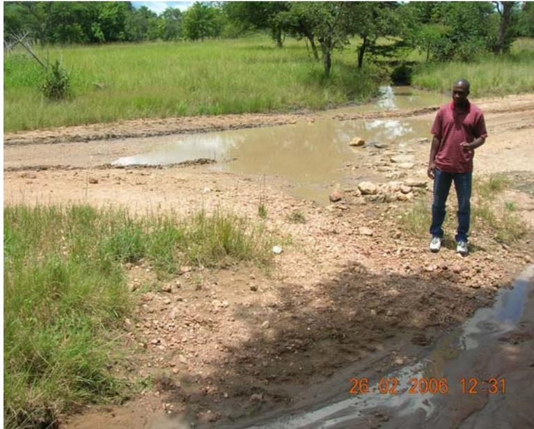
*A Section of the Choma – Chitongo road with a blocked Culvert*
