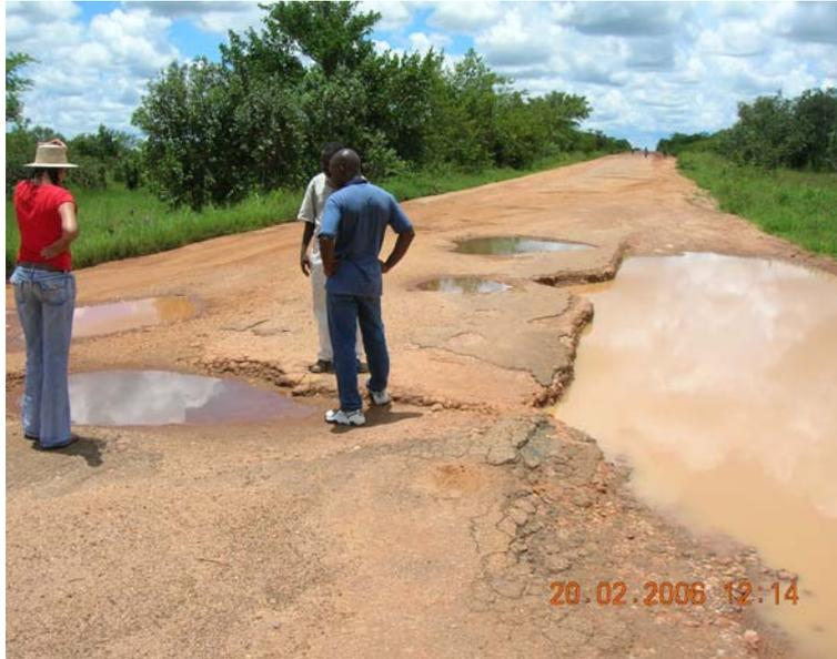
*LOT 2- Some parts of the road completely damaged and cannot support any layer of Tarmac.*
