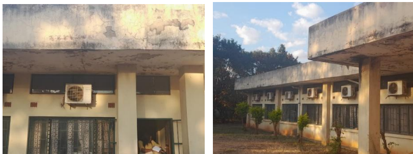
Old un-rehabilitated building occupied by officers
