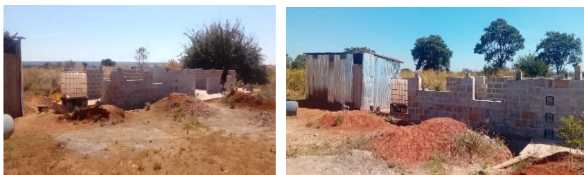
Construction works in progress at Misundu Milk Collection Centre in Ndola
