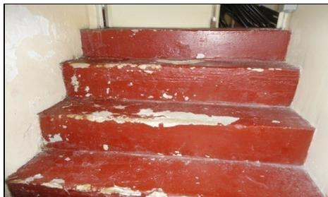
*Cracked Stairs leading to the basement*
