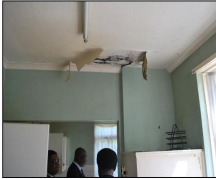
*Damaged leaking ceiling*
