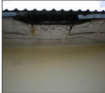
*Ceiling falling due to leaking roof at 6 Tshiniama Avenue*
