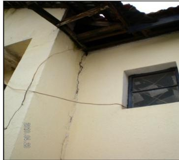
*Cracked wall and damaged roof at 6 Lundula Avenue*
