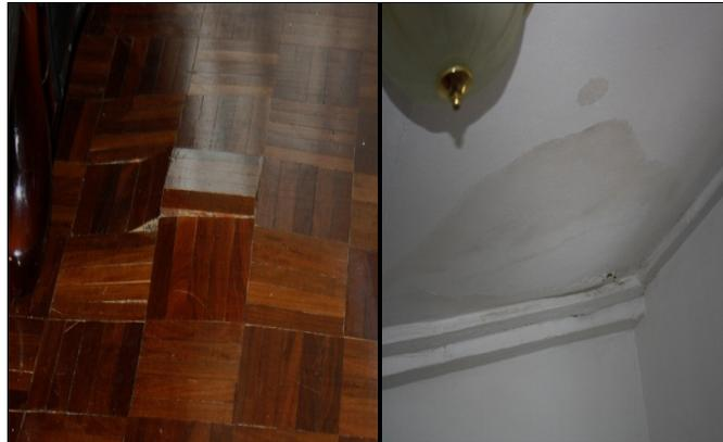
*Wooden floor tiles coming off    Damaged ceiling board*
