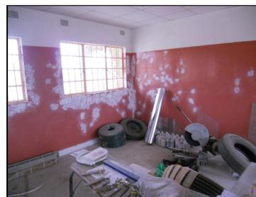
*One of the classrooms showing terra coat paint rejected by the engineer*
