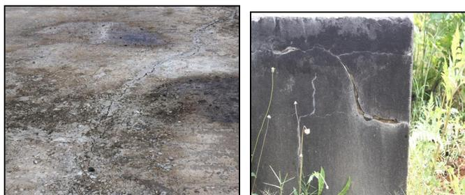
*Cracks in the substructure*
