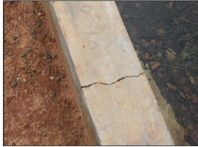
*One of the cracks on the culvert headwall*
