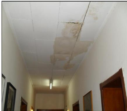
*Damaged ceiling as a result of the leaking roof at the Chancery*
