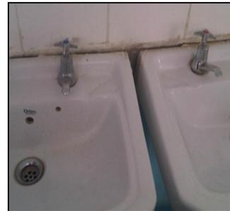
*Poorly fitted hand wash basins*
