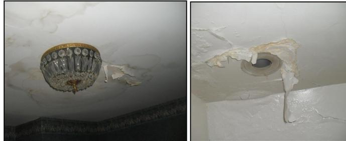
*Damaged ceiling board due to leakages*
