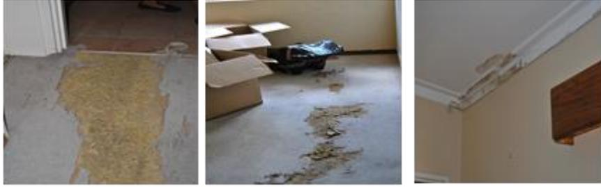
*Damaged carpet and leaking ceiling board*
