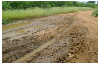
*Water ponding and Wheel ruts formed at 6.9km*
