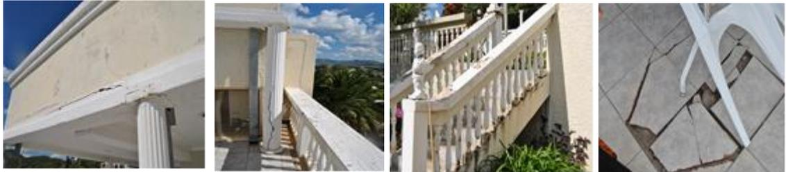
*Cracked pillars, outside walls, stairs and the damaged tiles in the Guest wing*
