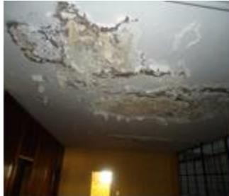
*Damaged ceiling due to roof leakages*
