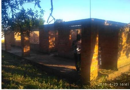
*Uncompleted office block at wall plate level*
