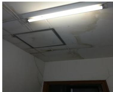
*Stained ceiling and Visible Cracks*
