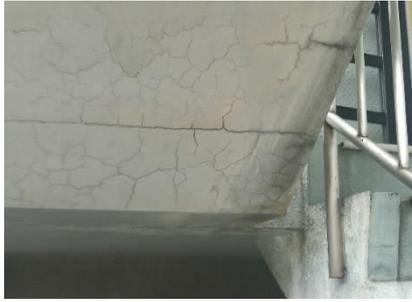
*Cracks under the Third Floor Stairway*
