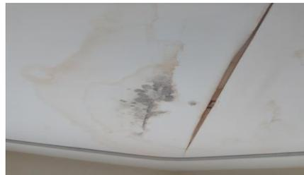
*Stained ceiling due leaking roof*
