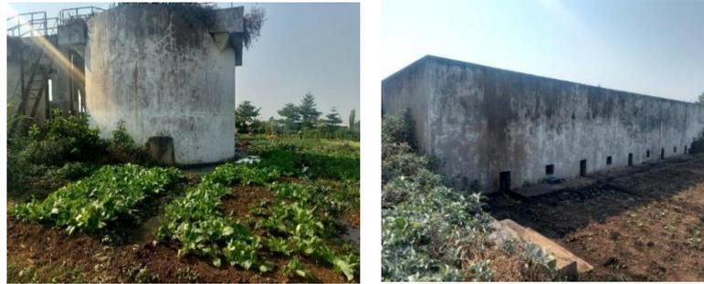
*Dilapidated Sediment Tanks with Non-Functional Filters*
