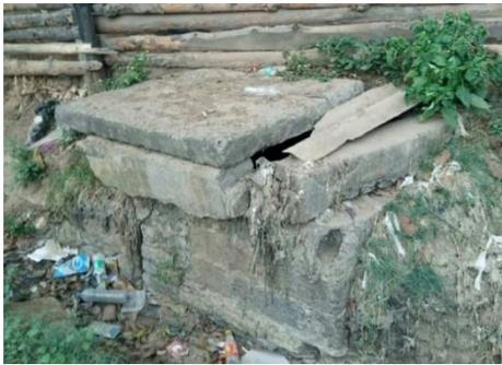
Poorly installed concrete cover on manhole
