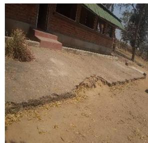
*Cracked slab and septic tank due to shoddy works by Pozzolona Enterprises*
