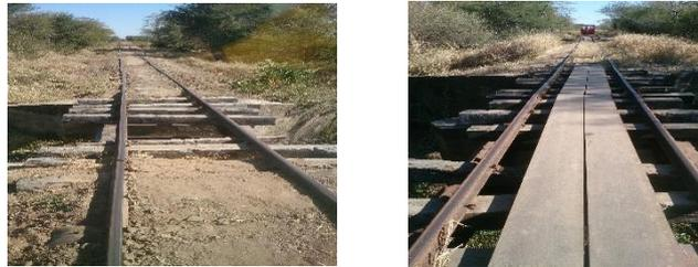
*Culverts with inadequate and misaligned sleepers – Mulobezi line*
