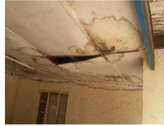
*Rotting ceiling board due to leaking roof*
