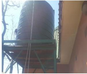
*Water tank erected too close to Ablution Bloc*
