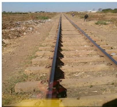
*Section between Lusaka and Kafue lacking ballast*
