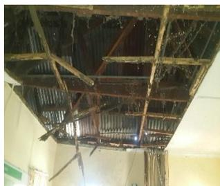
*Collapsed ceiling board*
