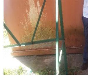
*Damaged ablution block walls due to water from the tank*
