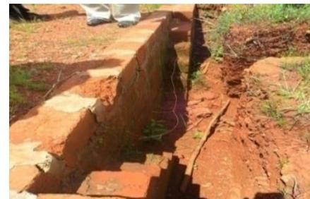
*Collapsed foundation walls as of September 2012*
